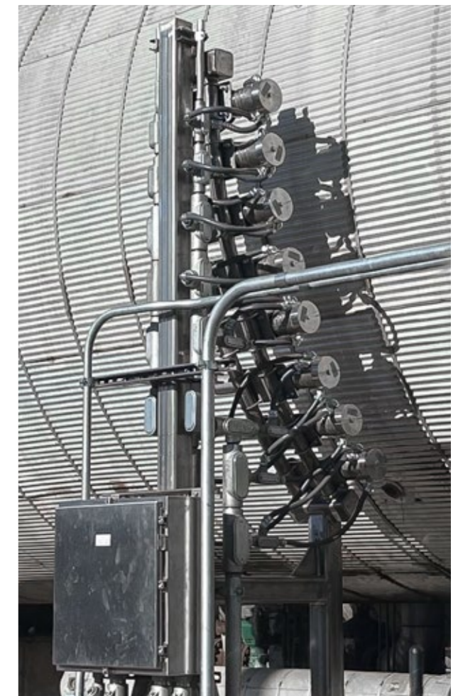
Fig.2 Berthold's EmulsionSENS mounted outside a desalter
